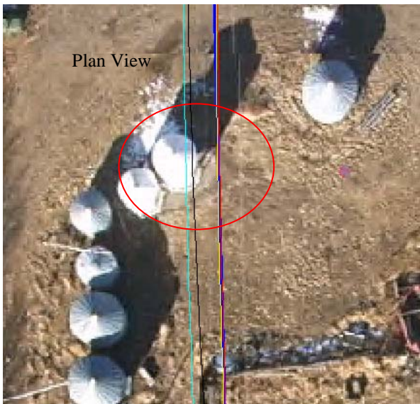
Fig. 7. 138 KV transmission line encroachments to silos.
